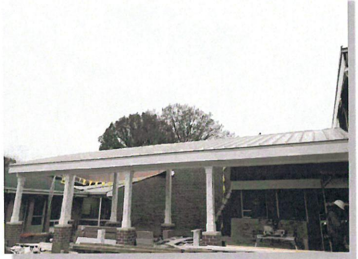
Standing Seam Metal Roof
