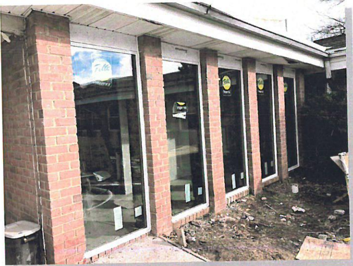
Kitchen Expansion Windows
