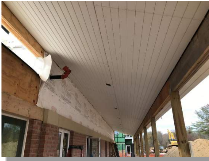
Commons Front Entrance Bead Board Ceiling
