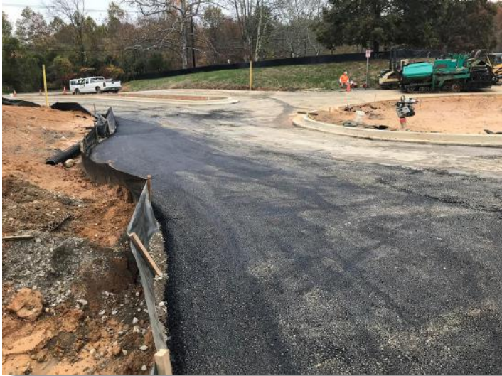
Base and Final Paving Main Entrance
