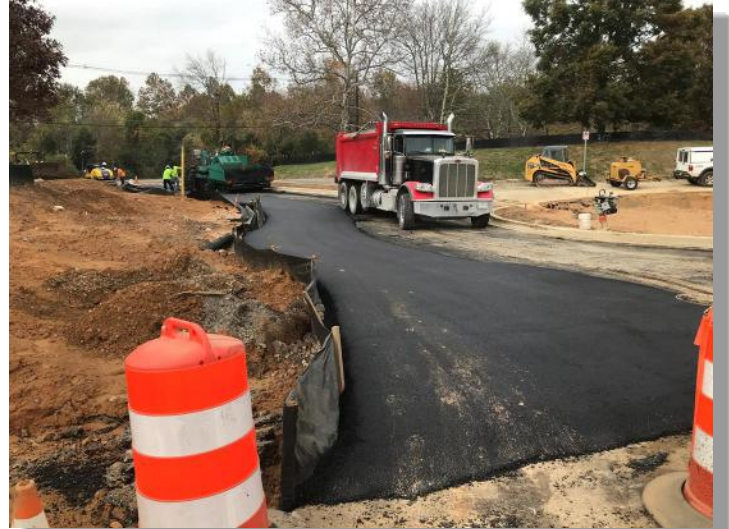
Base and Final Paving Main Entrance
