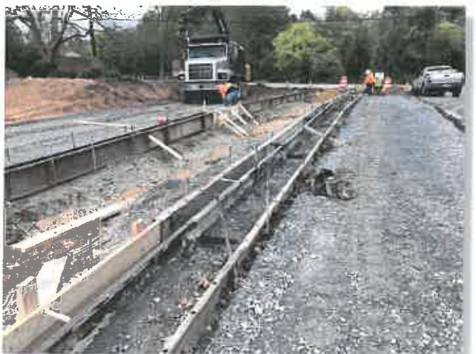
Main Entrance Road & Curb
