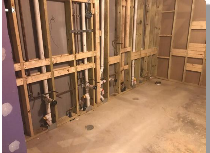
Men's bathroom plumbing rough-in
