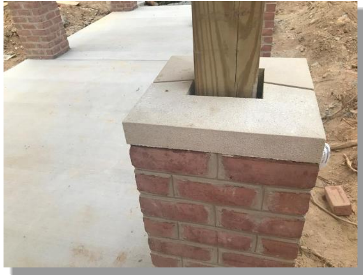
Brick columns at front entrance
