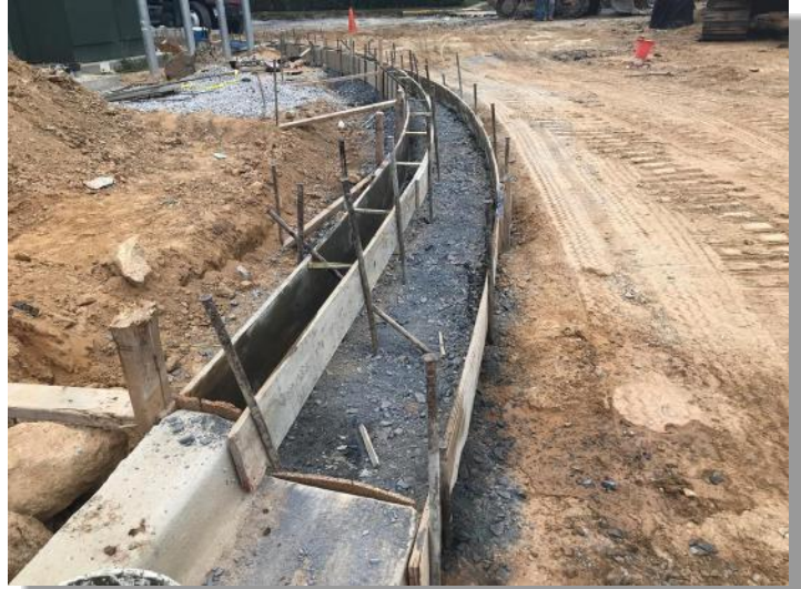
Curbs at the rear of Commons
